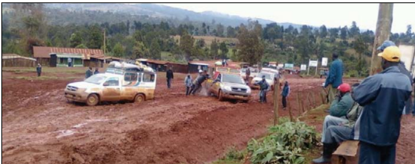
The deplorable state of the Iten-Kapsowar road during the rainy season in Elgeyo-Marakwet County
