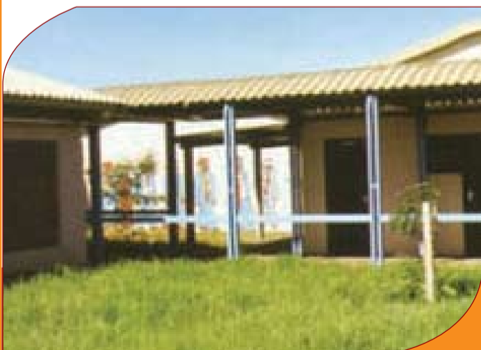
Isiolo District Hospital
