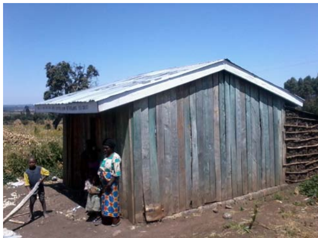
One of the small houses constructed by the KRCS in Burnt Forest
