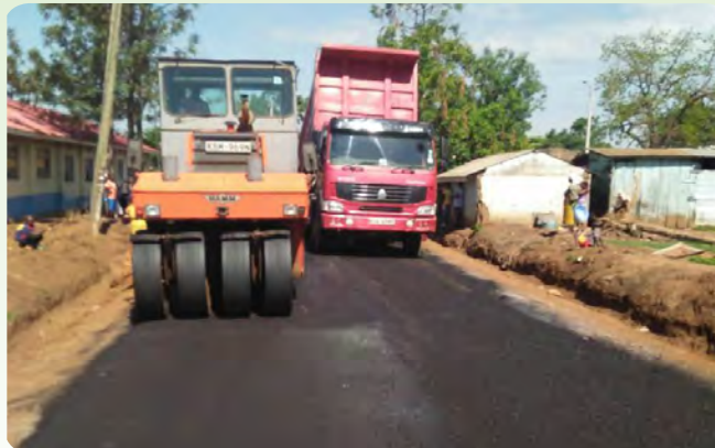
Ongoing tarmacking of feeder roads in Busia and Malaba towns
