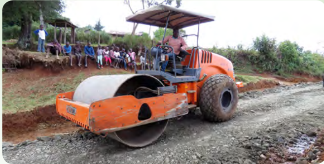
Ongoing gravelling and compacting of Lessos road in Nandi Hills Constituency
