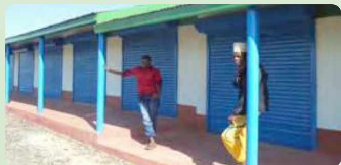
One of the 14 market stalls with 20 stalls each constructed in all the wards
