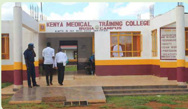
The newly constructed KMTCC, Busia
