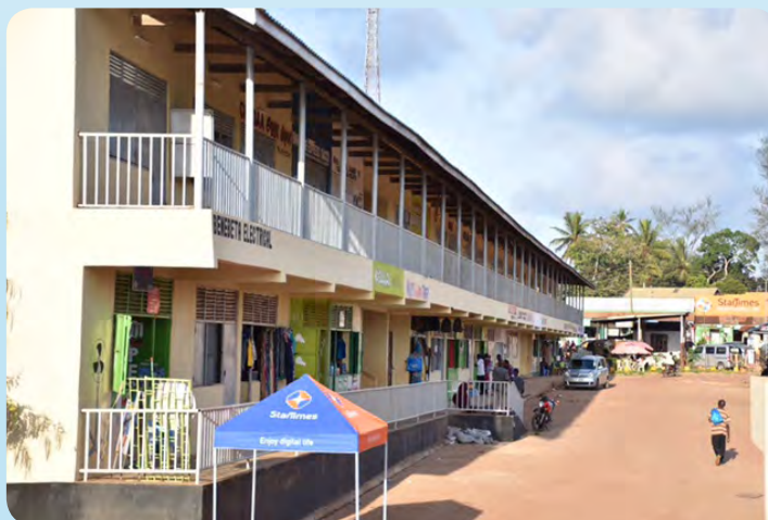
The Kwale Market stalls constructed by the County Government.
