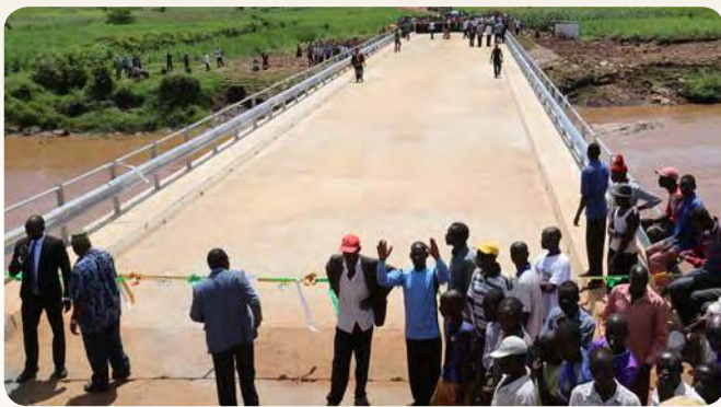
75 meter long Khaunga bridge built to the highest engineering standards
