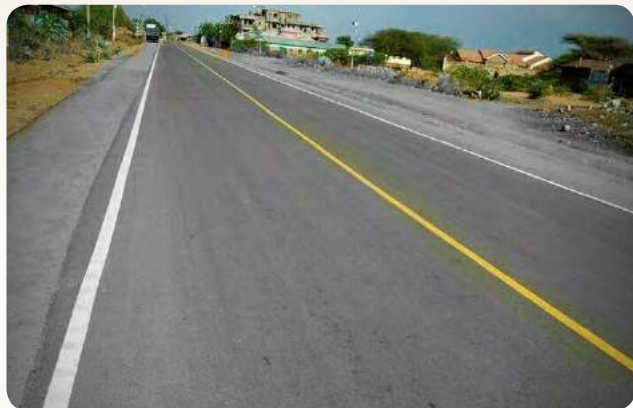
A section of the 25km tarmac road by Mandera County Government.
