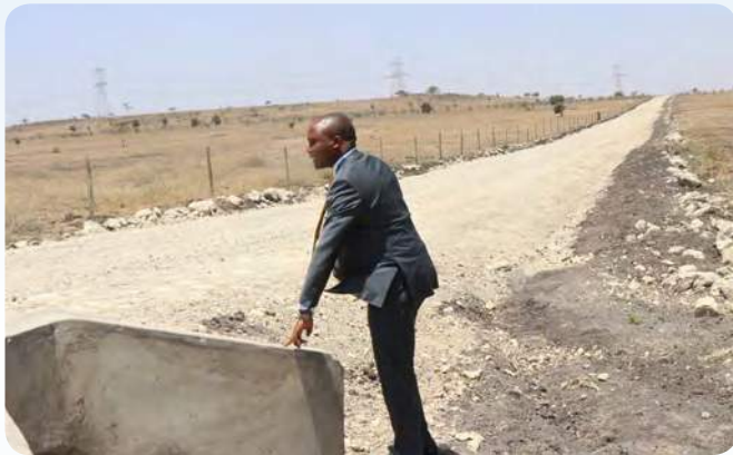
Kajiado CEC Alex Kilowua inspect rehabilitated Oloika - Matali road in Kitengela, Kajiado East Sub County
