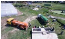
Decentralised Waste Water Treatment Facility (DTF), Nakuru County (Urban investments)
