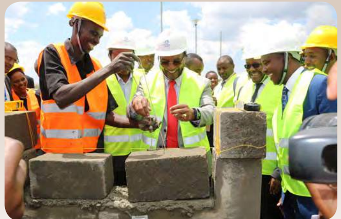
His Excellency Governor Francis T. Kimemia breaks ground for the new County Assembly offices in Ol'Kalou.
