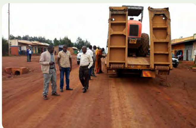
Part of the Brigadier-Misikhu Road under construction
