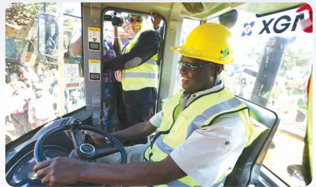
Governor Kiraitu flags off the road construction works at Gitimbine
