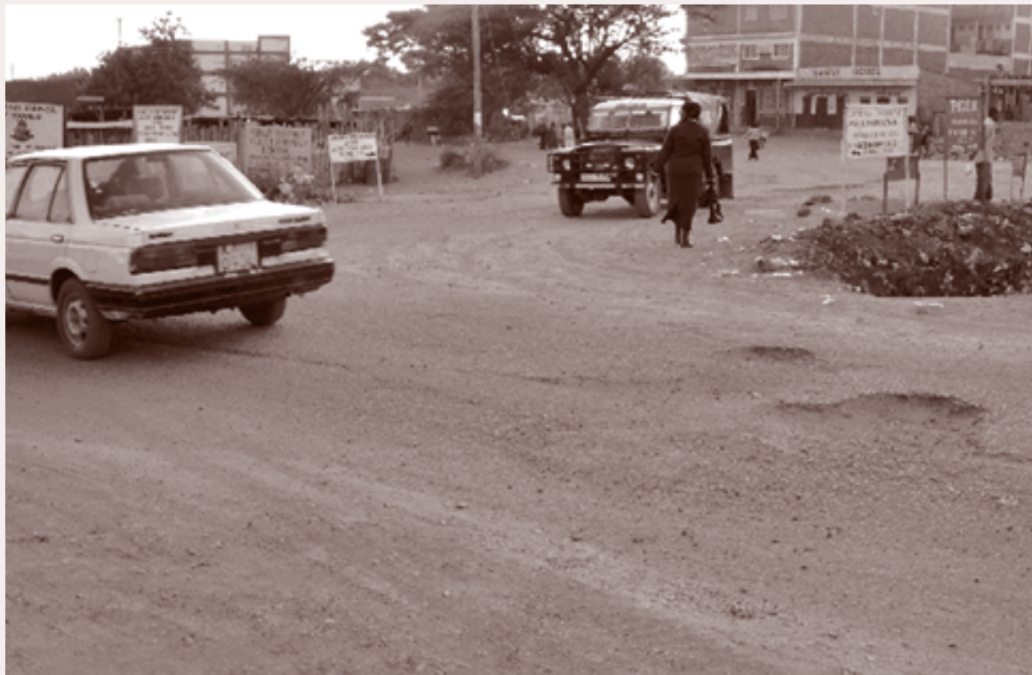
"Bad roads and under development in Isiolo"
