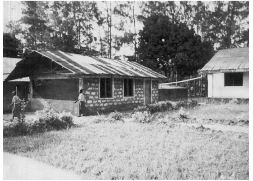
Mwaumba primary school which will be demolished
